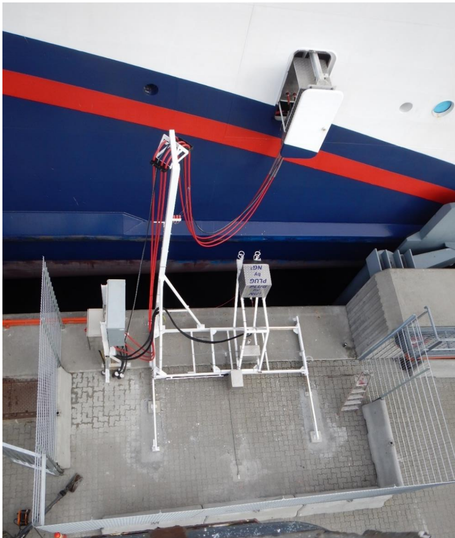
PLUG is light weight and avoids any significant harbour engineering when vessels are docking alongside the quay
